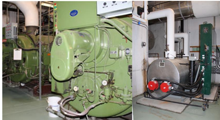
Image 3 The University's hybrid heating systems uses electricity for heating at off-peak times.
