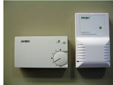
Occupancy sensor driven temperature Setbacks
