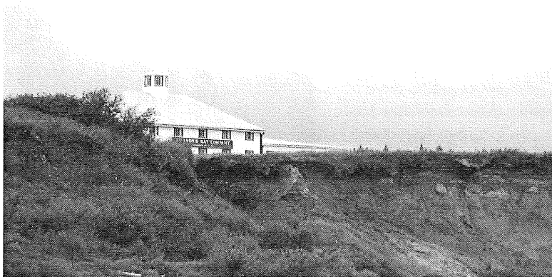
Slumping river banks threaten the historic depot building at York Factory NHS. See article on page 13 for more details.
