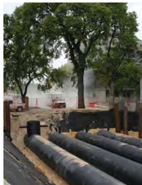
Cisterns installed deep beneath Richardson Green Corridor in August 2011
