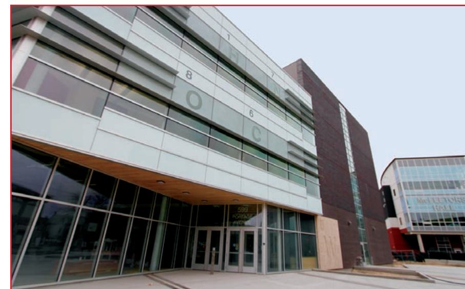
The new Richardson College for the Environment and Science Complex at Portage Avenue at Langside.
