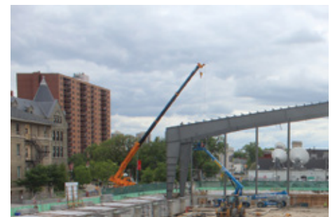
The UNITED Health & RecPlex is on track for completion by summer 2014. You can watch this state-of-the-art facility take shape in real time via live webcam at uwinnipeg.ca/recplex-live
